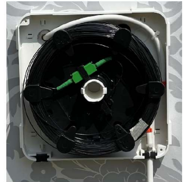
Midi-ITB shown with coil, 7/4mm LSZH MD fitted with ELF restraints – above.
